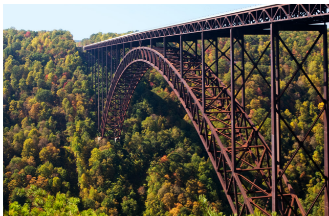
Weathering Steel Bridge
